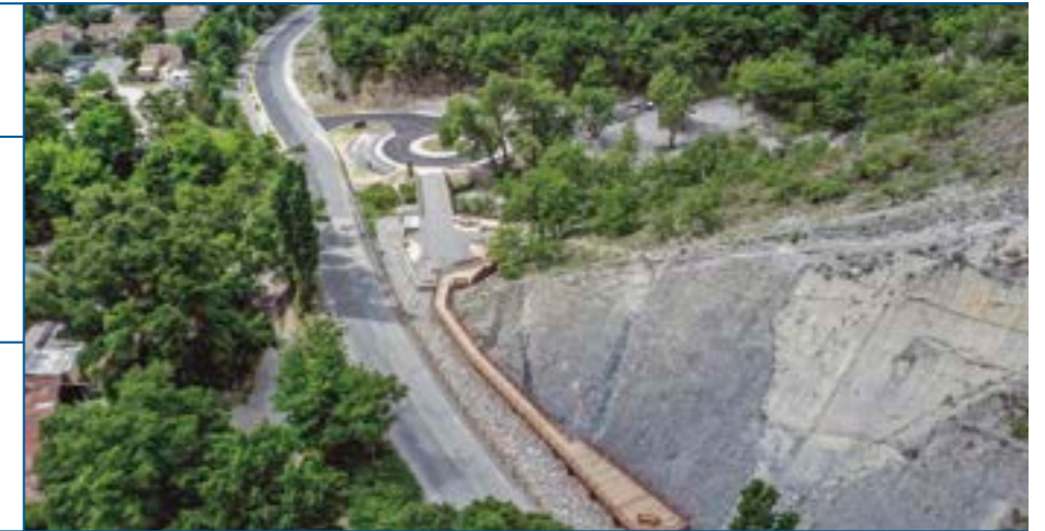
Drone view showing the site facilities: visitors' path, mediation area, footbridge accessible to people with reduced mobility, and observation platform. (@Haute-Provence Global Geopark).
