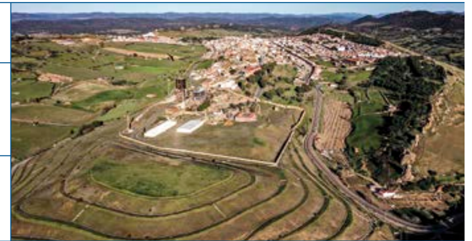
General view of the town of Almadén, Spain, in the foreground are the mercury mining facilities located to the west of the town and in which the main shaft and their metallurgical fence stand out.
