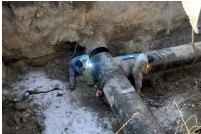
Figure 9.8. Repair work of water network of Van City (from Van Municipality, 2011).
