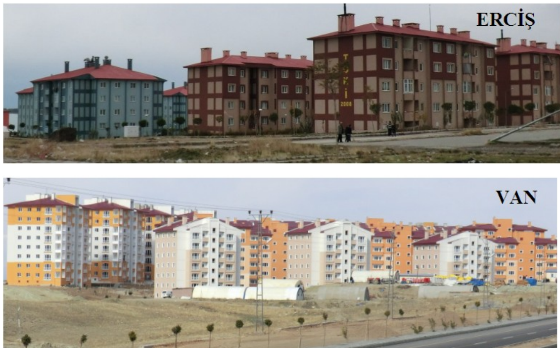
Figure 7.4. Views of non-damaged TOKİ buildings.
