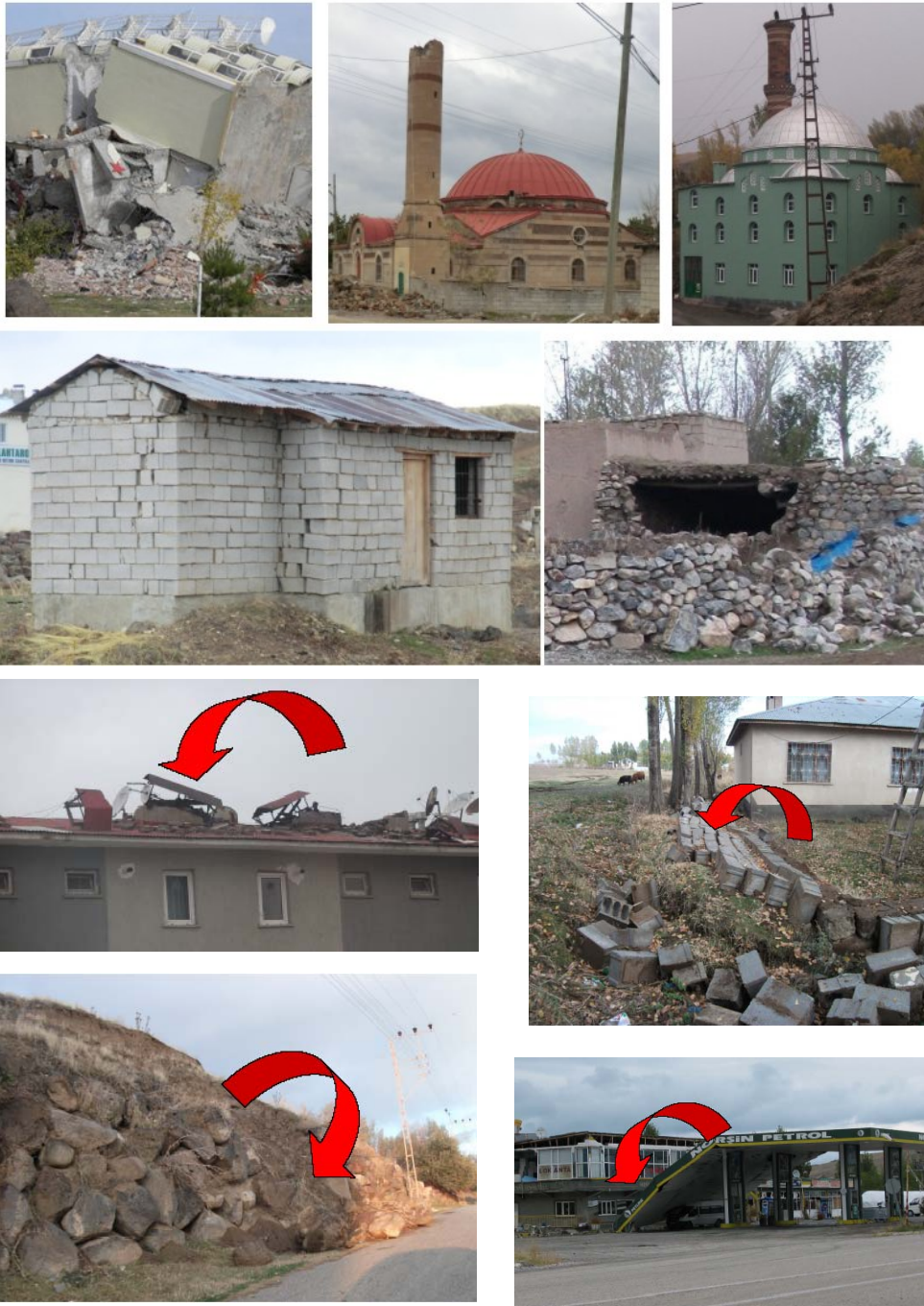
Figure 6.13. Views of failed, toppled and displaced some structures in the epicentral area
