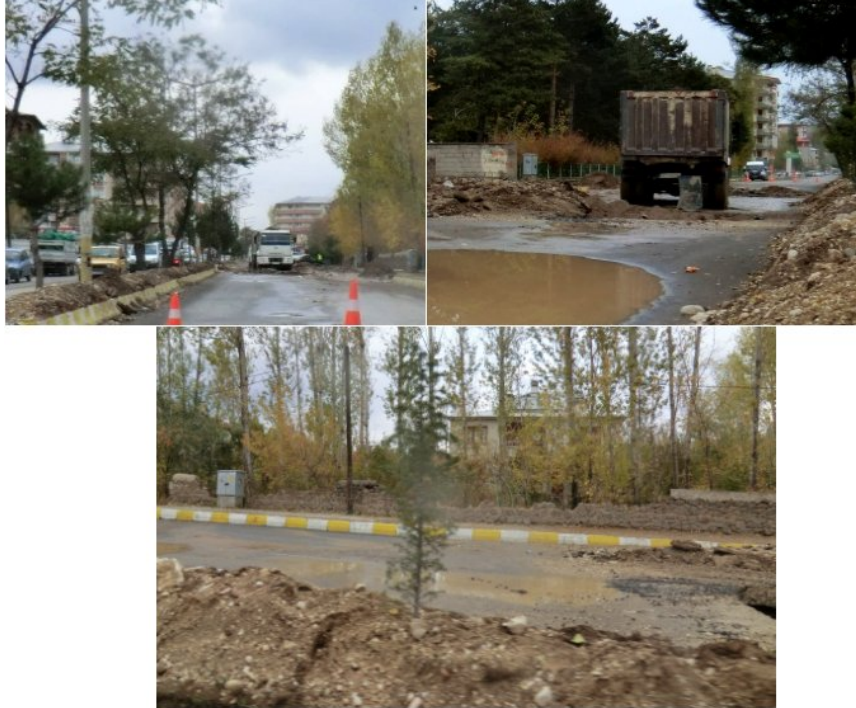
Figure 9.12 Repair work of sewage in Erciş
