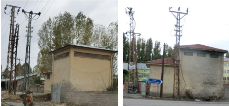
Figure 9.3. Non-damaged sub-stations in Erciş.
