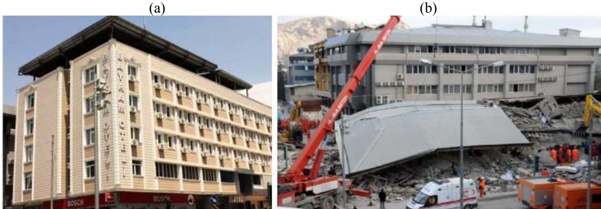
Figure 11.9. Views of Bayram Otel (a) before and (b) after the Van-Edremit earthquake (Anadolu Ajansı, 2011).
