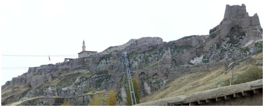
Figure 7.20. A view of Van Castle after the earthquake.
