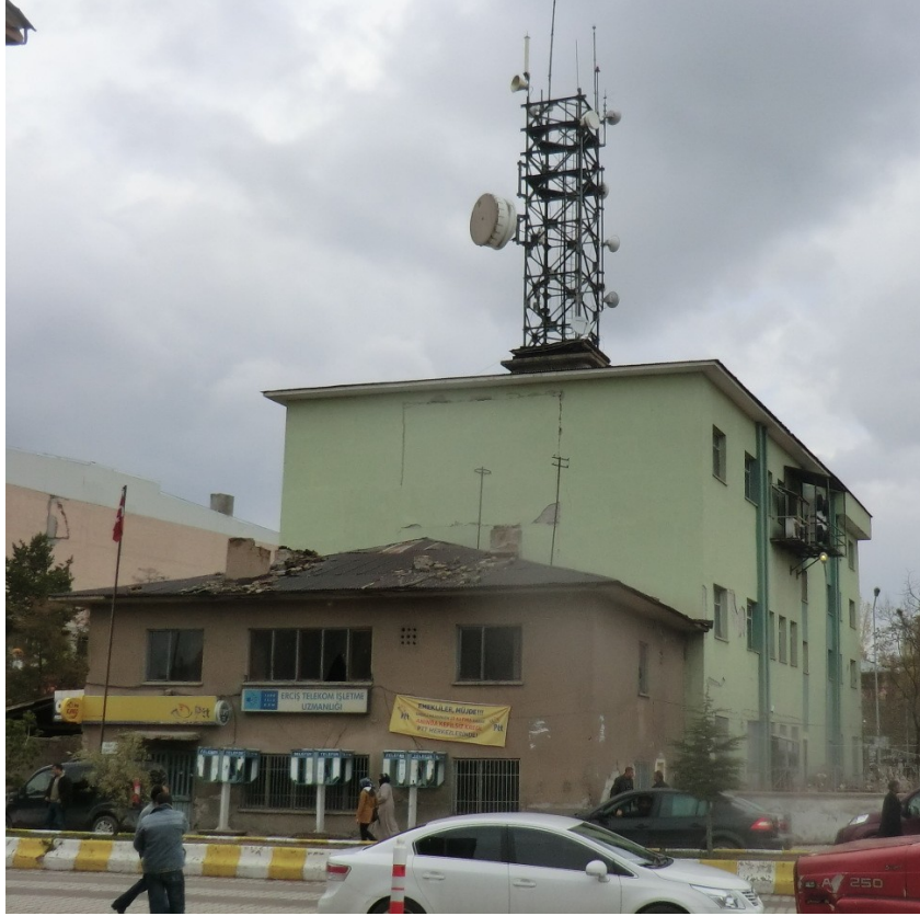
Figure 9.13. Slightly damaged main building of the TÜRK-TELEKOM in Erciş.
