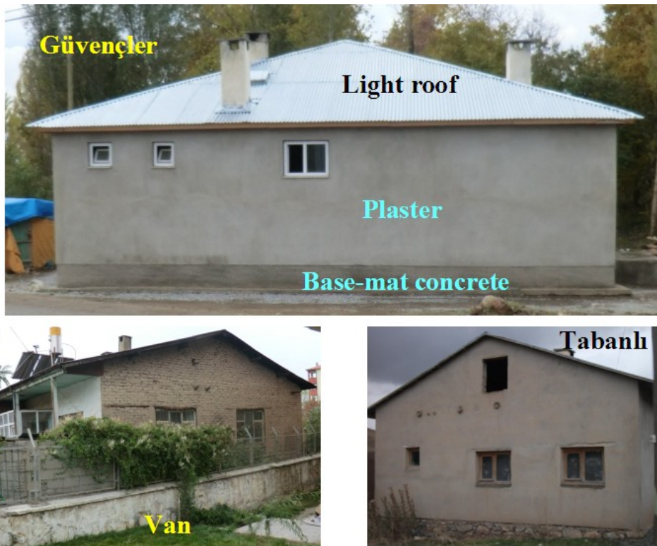
Figure 7.9. Views of non- or slightly-damaged masonry buildings in several localities.
