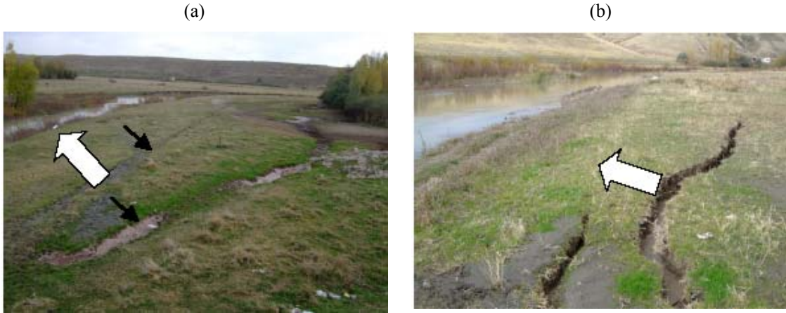
Figure 10.22. Lateral spreading cracks parallel to Evlangaz Stream; (a) Topraktaş village and (b) near the road between Topraktaş and Arısu.
