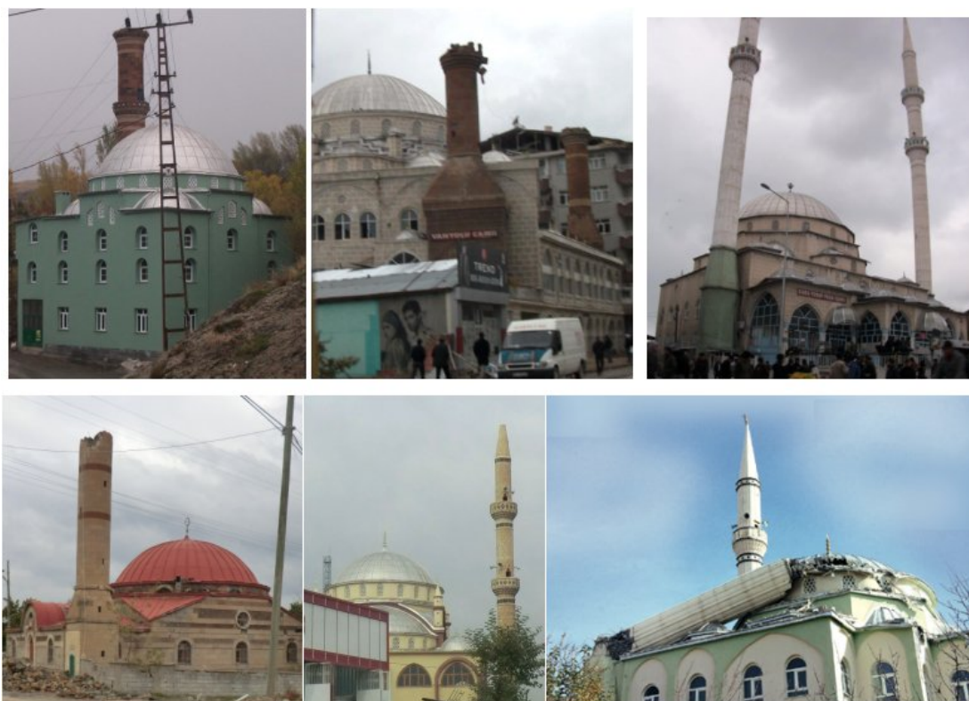
Figure 7.1. Views from damage to mosques and their minarets.
