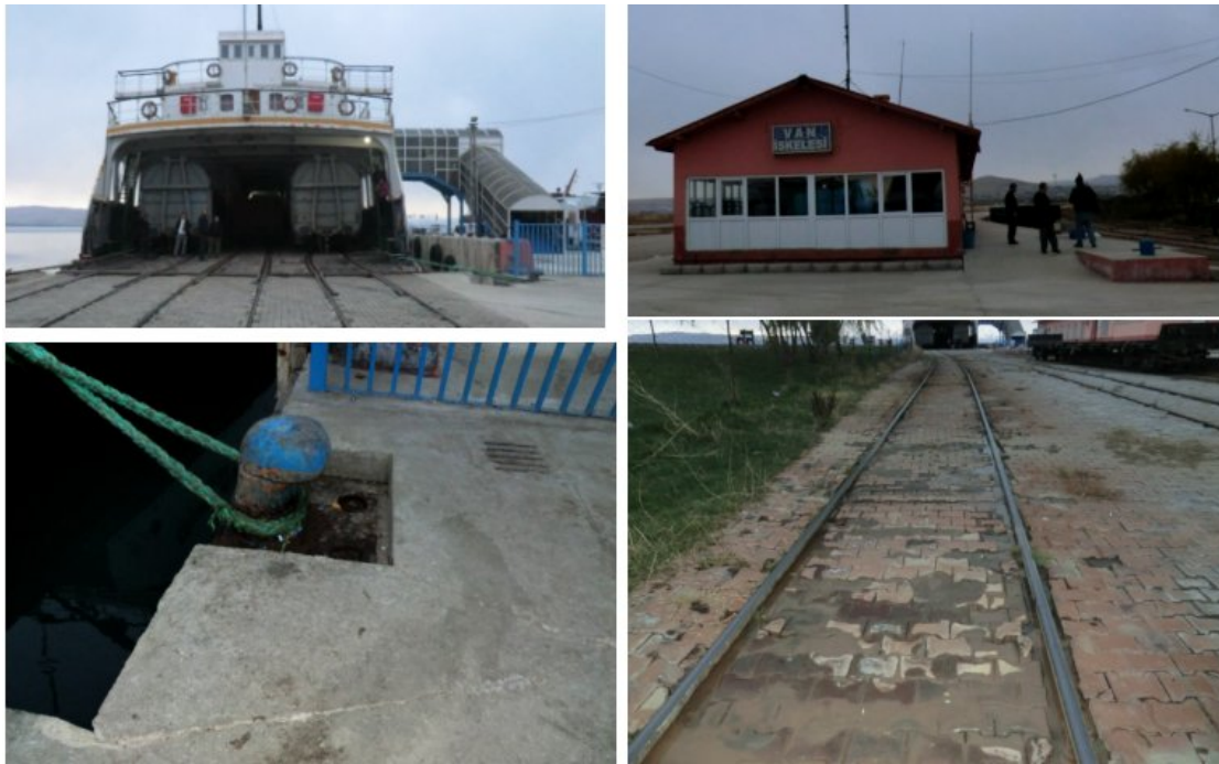
Figure 8.11. Views of slightly damaged Van Port.
